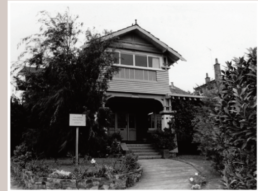
Lindsay Field House at 21 Aberdeen Street, Geelong, was home to the Geelong branch from 1980 until 1985. It was named after the Lindsay Field Trust, which donated most of the money to purchase the property.
